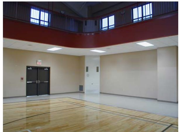
Two of eight corner consoles units located in gymnasium, one on lower level and one on upper level
